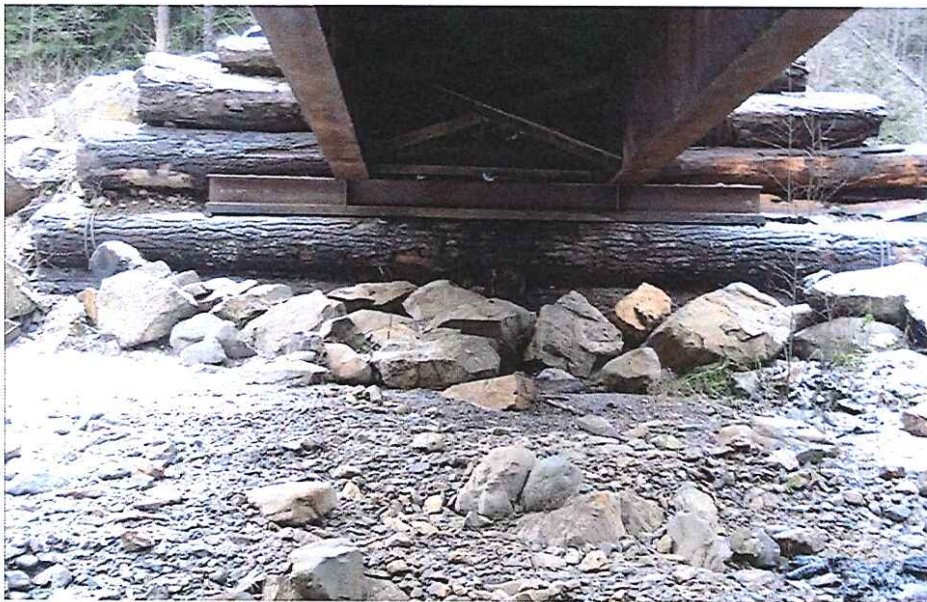
CK2237 Left Abutment
