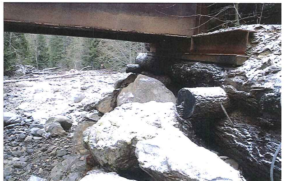
CK2237 Right Abutment
